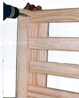
FASTENING RAIL FROM THE INSIDE
